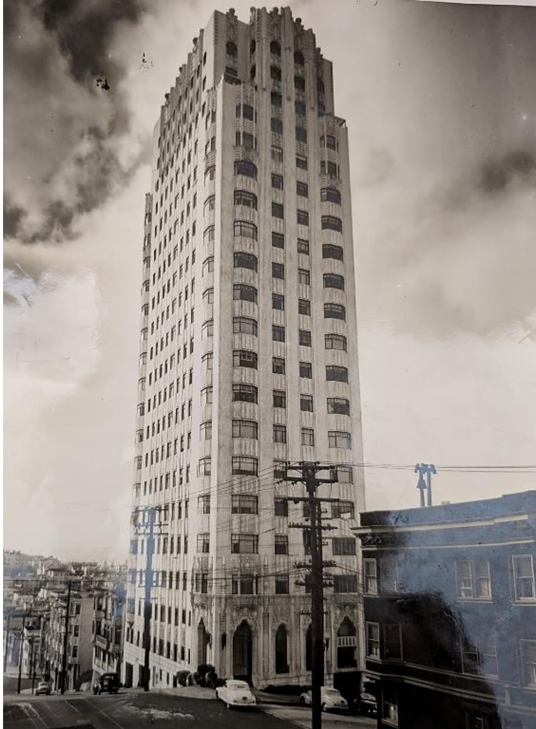
Figure 4 Assessor photograph of east (left) and north (right) elevations, September 1944; Source: San Francisco Public Library, History Center
